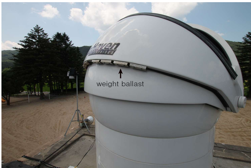
Figure 3. Equip the eight of 2kg weight ballast of each shell to allow fully automatic opening and closing.
